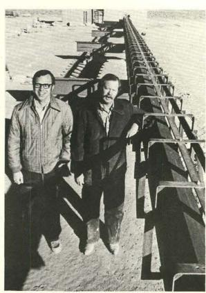
ROCKET SLED track at TTR used for the tornado safety studies is constructed from steel I-beams with welded safety cage. At left is project leader Al Stephenson with Jack Windsor (both 9473).
